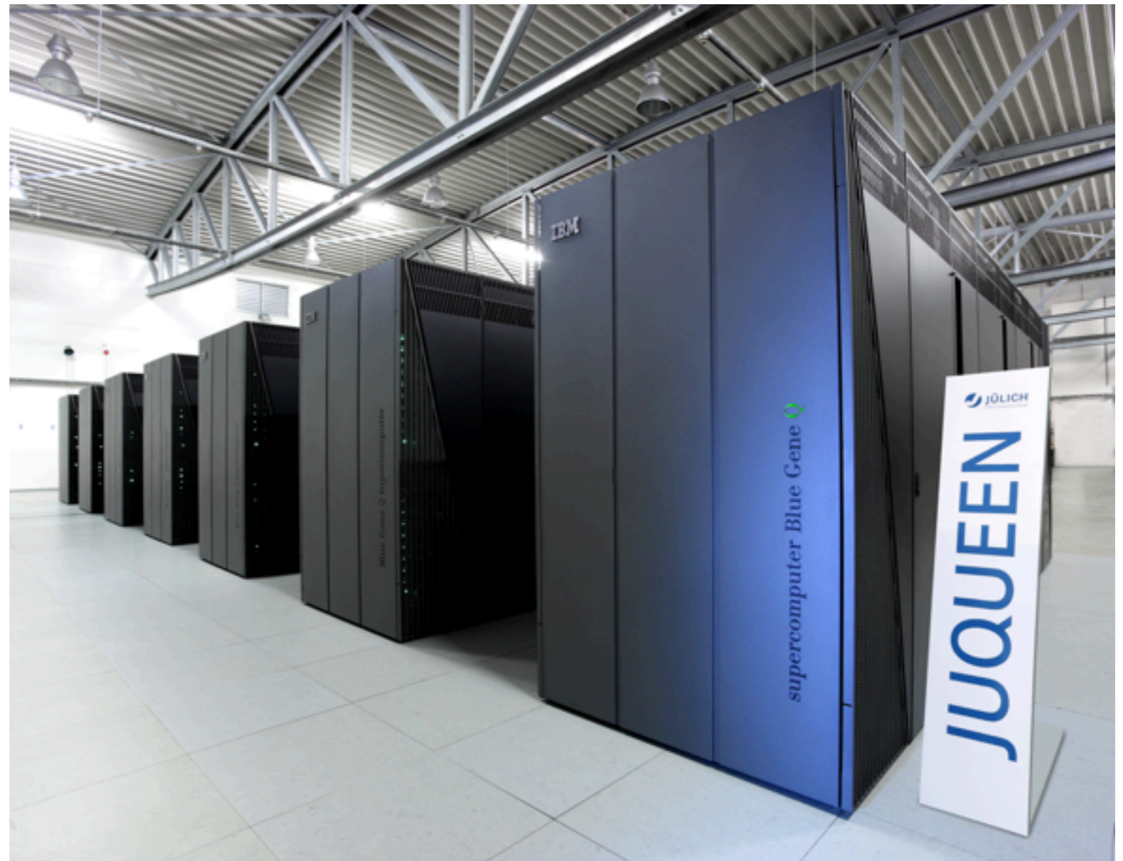
Figure courtesy of Jülich Supercomputer Centre (JSC)
